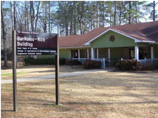
Conference Center at Rock Eagle 4-H Camp, Eatonton, GA.
